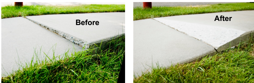
Figure 7: Precision Sidewalk Safety Work Example
